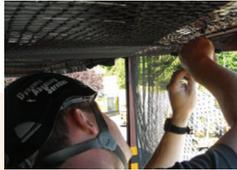
Netting is one of the most popular and cost effective. Can be used to protect a very wide range of structures, plant, equipment, voids, ledges, shop canopies and complete roof areas. Special flexible net frames are also available to support nets away from features such as statues, lights, decorative items and signs.
