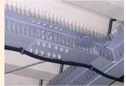
Bird spikes are the simplest and most cost effective solution for deterring seagulls, pigeons and starlings in low-pressure areas. Special clips are available for installation to windows, gutters and beams.
