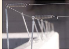
The wire system involves thin sprung wires mounted on posts just above the building surface, well suited to ledges, beams, parapets, gutters and roof ridges. A very adaptable and discreet system used widely.
